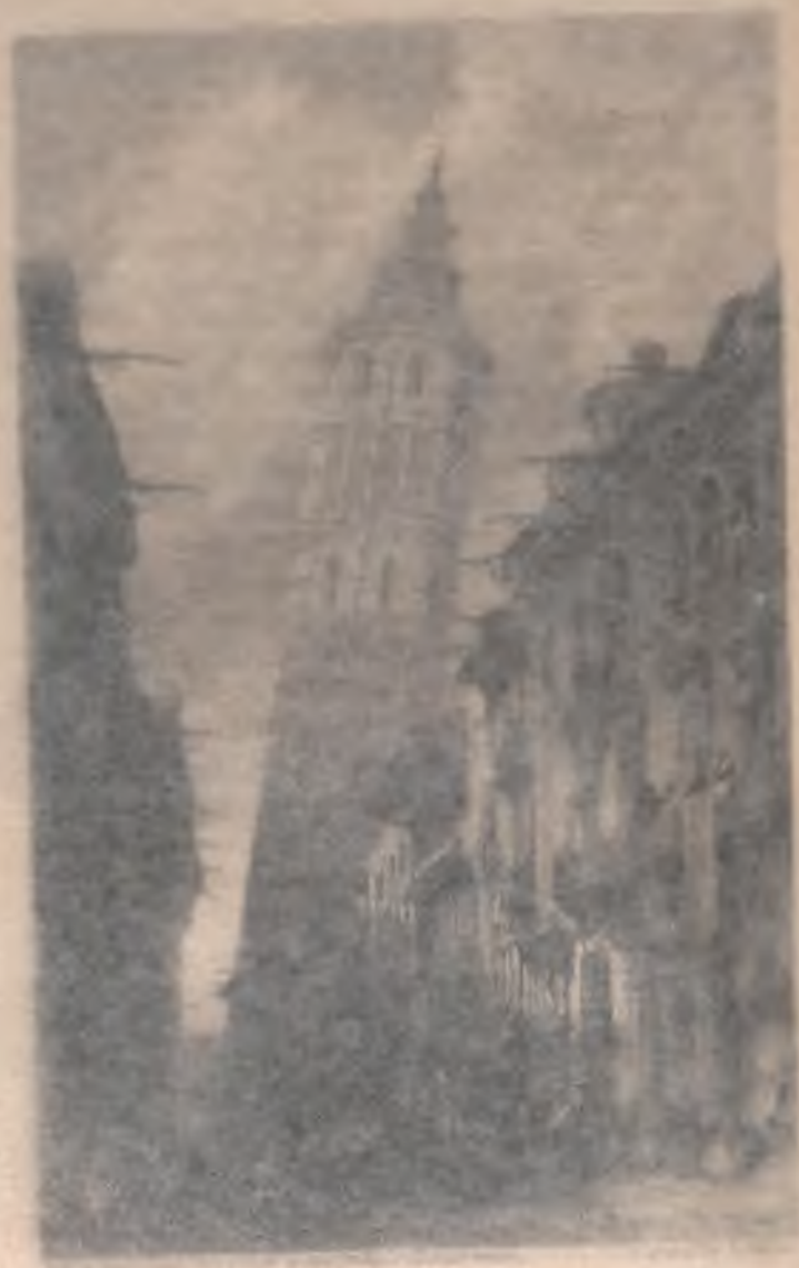
LEANING TOWER OF SARAGOSSA.
